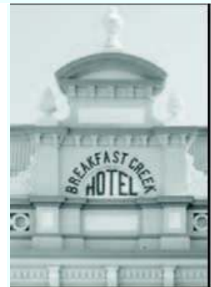
Woollam Constructions played an integral role in developing the original Breakfast Creek Hotel.
